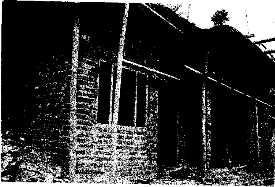
Fig. 3 Clay brick masonry house under construction. Note lintel band and gci sheets for placing the concrete slab.
