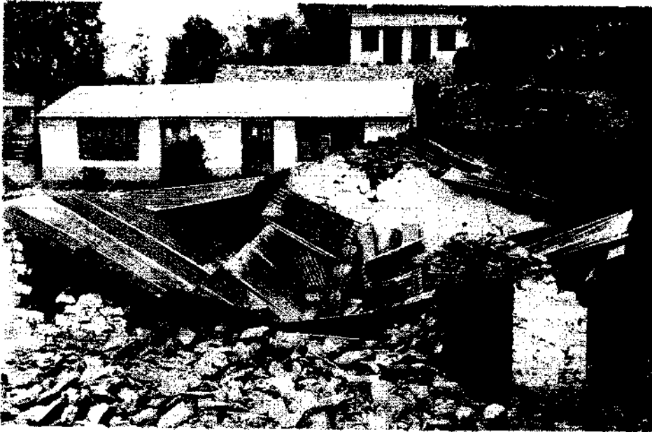
Fig. 14 Total collapse of roof due to out-of-plane failure of supporting wall and the roof supporting structure (school building, Bairagana).
