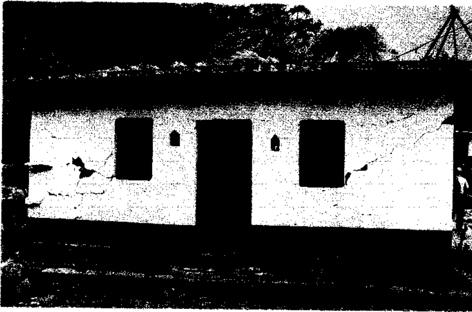
Fig. 13 Diagonal and x type shear cracks in newly built stone masonry house.
