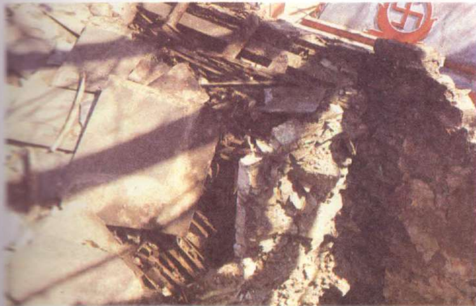
Fig. 21 Damaged house in Pipalkoti
