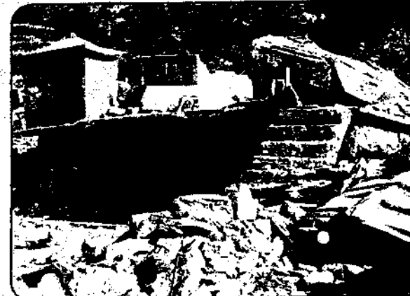
Photo 70 Collapse of first floor of a house in Byala Tipri village with deep open cracks in the ground and first floor. (New construction).
