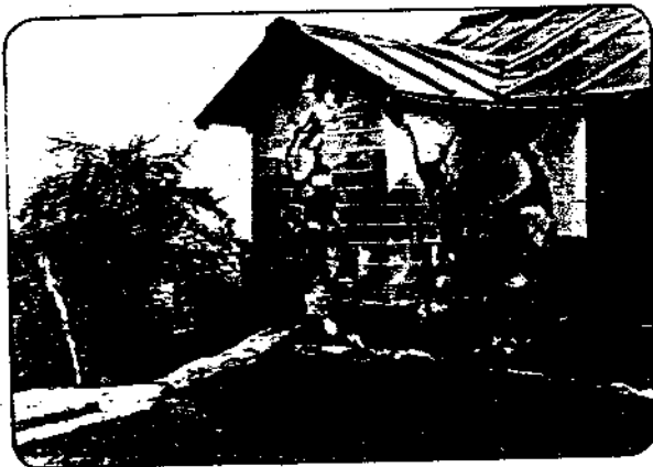
Photo 84 Damaged residence of doctor in Jakheli village.
