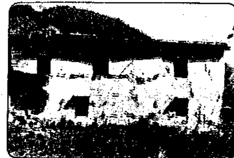
Photo 38 Collapse and cracks in the long walls of a house in Ganeshpur village.
