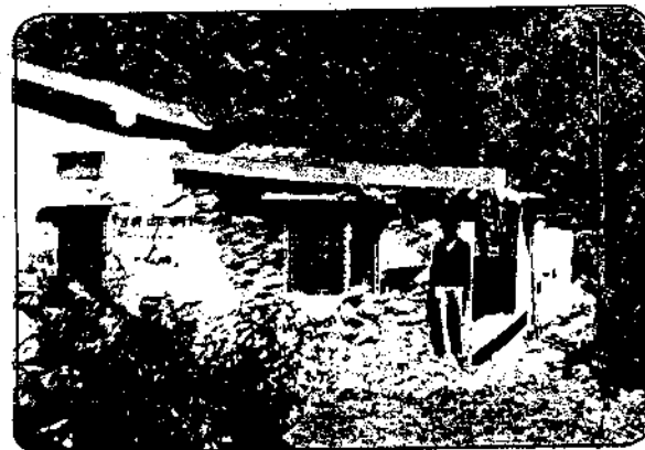
Photo 54 A Destruction of a cluster of type-A houses located on a N60°W-S60°E trending narrow ridge in Sanglai village.
