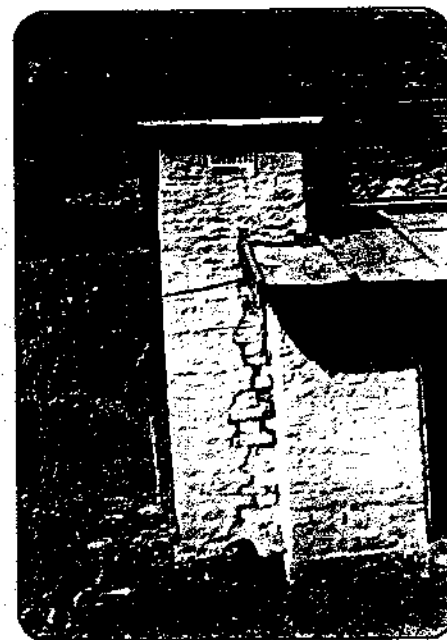
Photo 113 Separation and cracking of chimney in the out house of PWD Rest House, Gaurikund.
