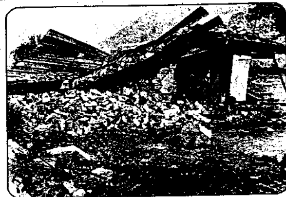
Photo 33 Complete collapse of a school building in Jakhol village.
