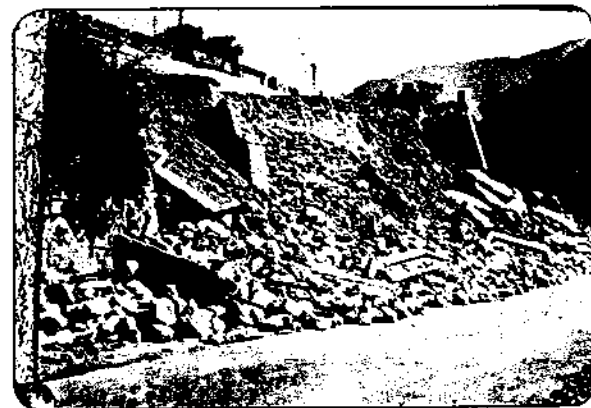
Photo 2 Failure of buttressed breast wall of the approach road to Maneri colony. (Photo NGRI).
