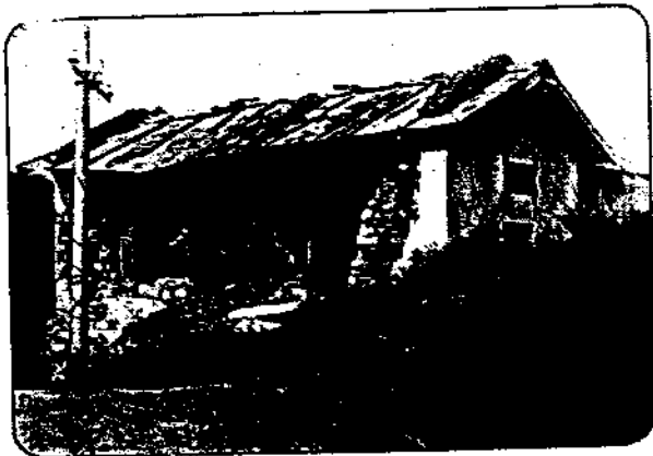
Photo 86 Collapsed veterinary hospital in Jakholi village.
