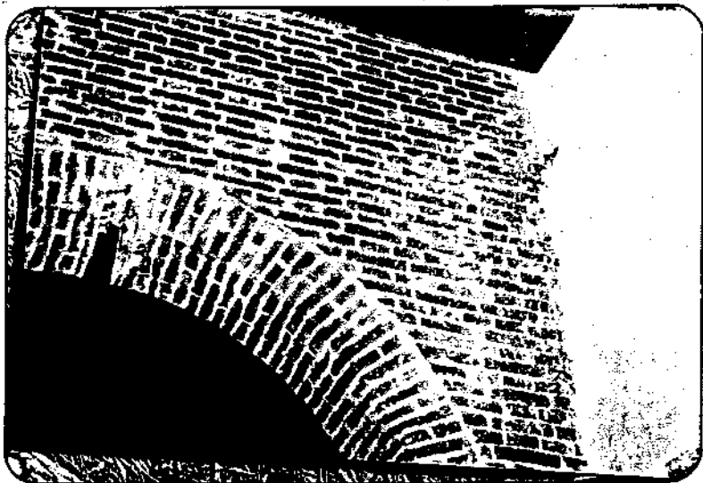
Photo 97 Dislodged brick from the centre of the arch portion of the first floor corridor-FRI building Dehradun.
