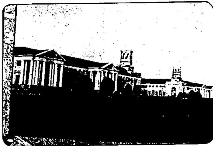
Photo 95 A general view of FRI building, Dehradun.
