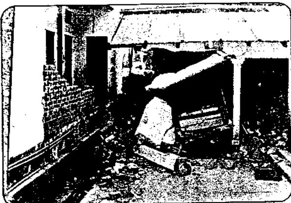
Photo 22 Collapse of pillar and beam of the verandah of a house in Police Lines, Uttarkashi.
