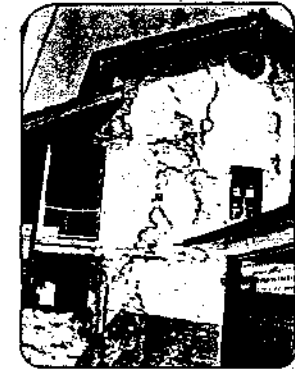
Photo 20 A A view of damages suffered by a conventional construction in Uttarkashi town. (Photo NGRI).
