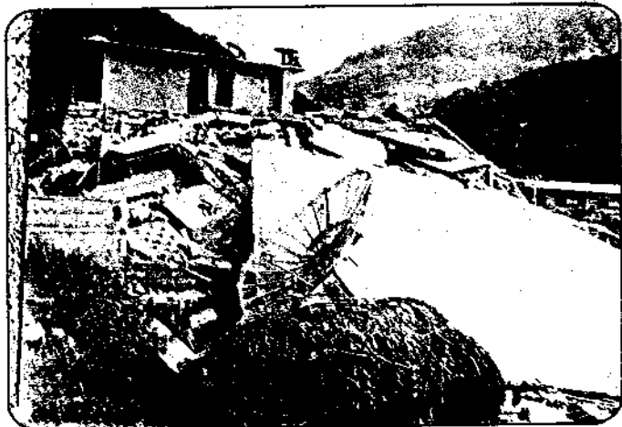
Photo 30 Complete collapse of a house with RCC roof at Aungi village. Note relatively much less damage in a house at the top left corner.
