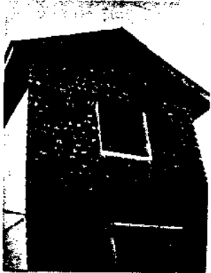
Photo 102 Bulging of the west wall of double storey Rest house at Chitkul.
